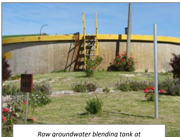
Raw groundwater blending tank at Softening Plant.
