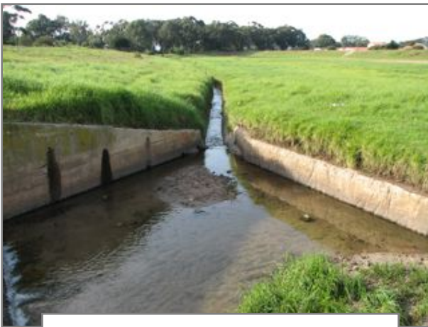
Basin 3: Storm water inlet.
