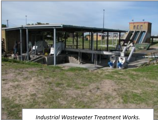
Industrial Wastewater Treatment Works.
