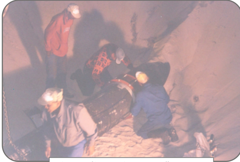
Night repair of burst pipe by AWRMS staff.
