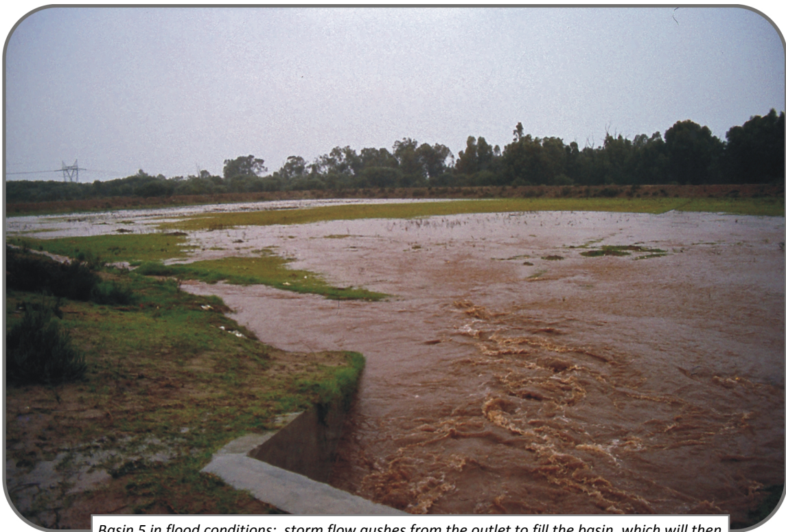
Basin 5 in flood conditions: storm flow gushes from the outlet to fill the basin, which will then drain away in dry weather.
