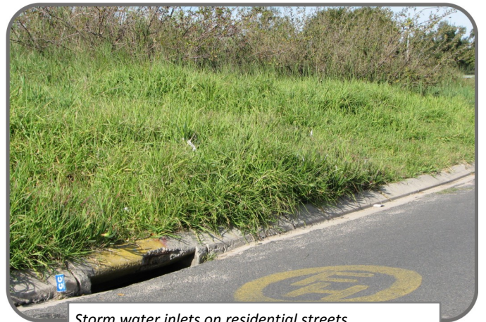
Storm water inlets on residential streets.
