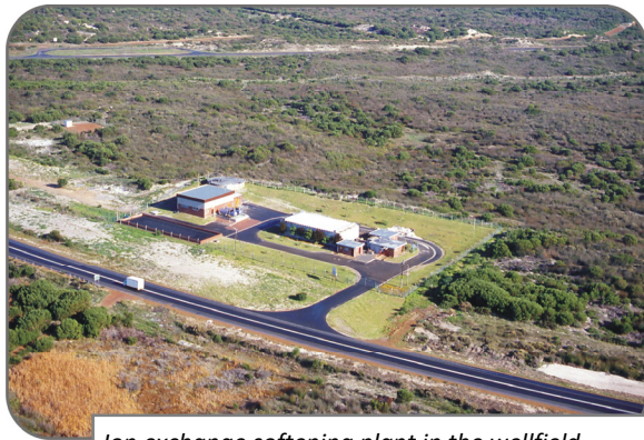
Ion exchange softening plant in the wellfield.
