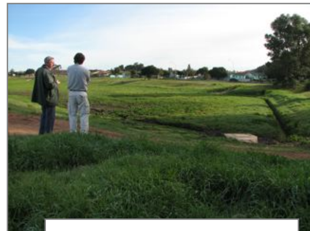
Basin 3: Storm water outlet.
