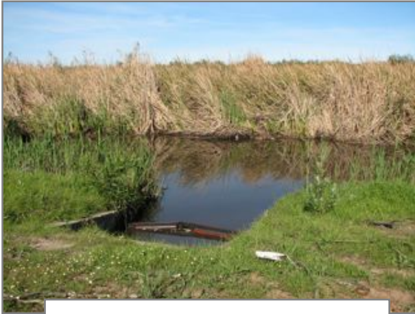
Basin 9: Industrial storm water detention.
